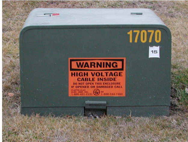
Padmounted Transformer
